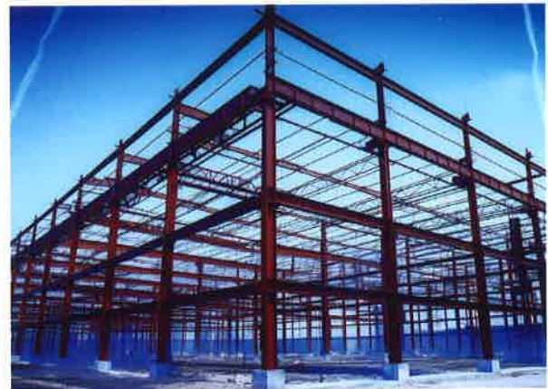
Steel structure industry
