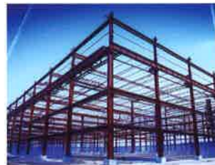
Steel structure industry
